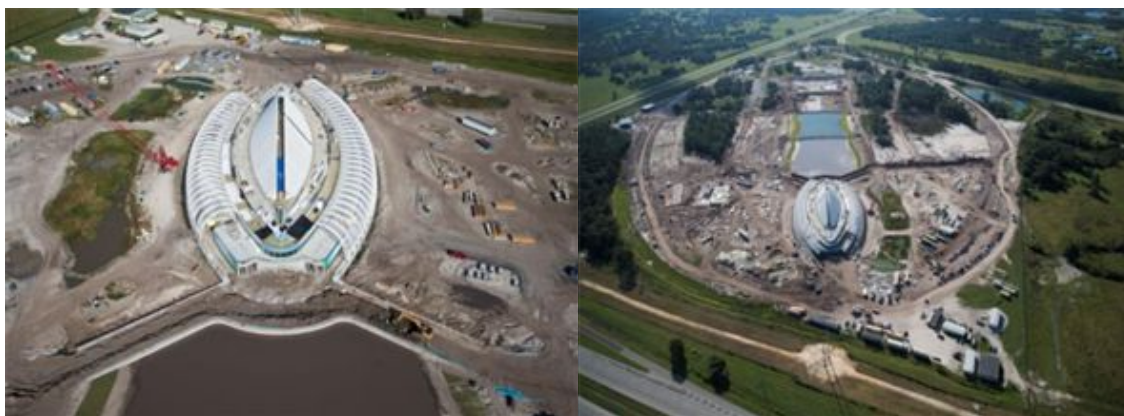
Innovation Science & Technology Building (October 2013)
