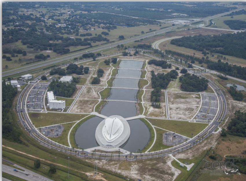
Florida Polytechnic University Campus View
