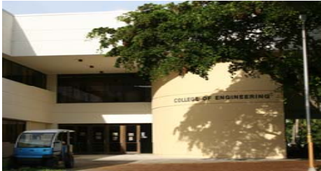
Engineering West – bldg. 36 59,000 GSF
